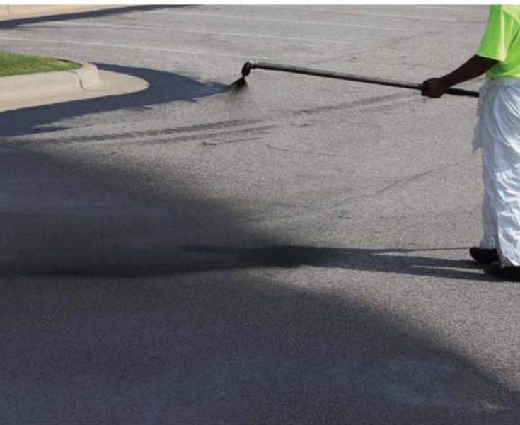
*Top:* Hand-spreading of sealant using a squeegee should occur in corners, edges and in confined areas.
